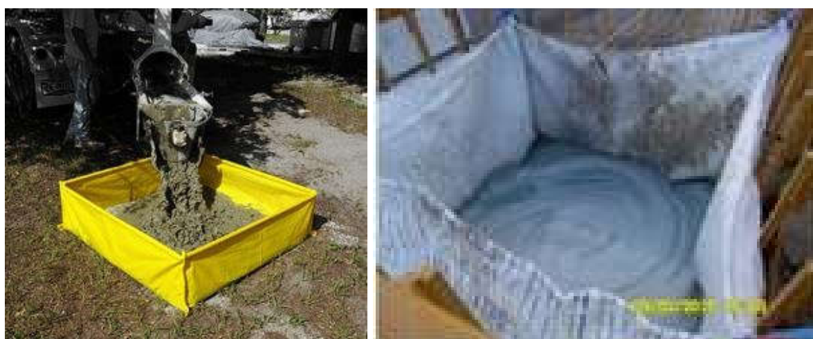
Plate 10.1 and Plate 10.2: Example Photos of Concrete Washout On Site Fuels and Chemicals
